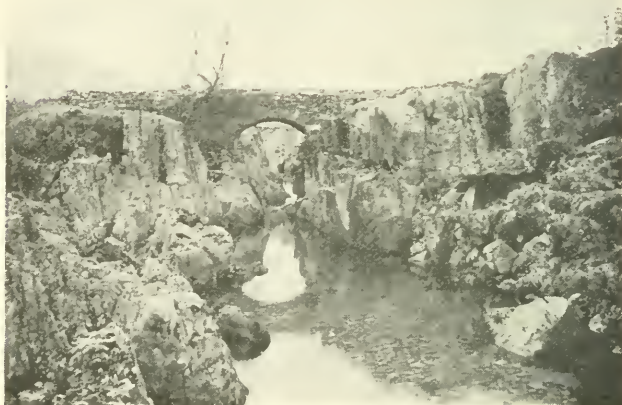
Birks Bridge over the Duddon
